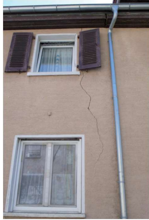
Figure A4.3.57. Cracking observed at connections between different building elements(left) and balustrade crack (right) caused by the 2014 Darmstadt earthquake. From Schwarz et al. (2015).
