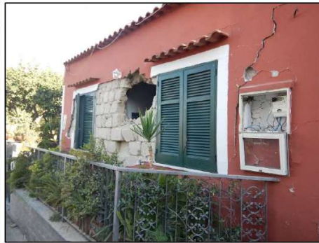
Figure A4.13.50. Out-of plane wall failure in Fango at Lacco Ameno (left); masonry expulsion and diagonal cracks in Casamicciola red zone (centre); delamination of wythes and corner failure (right). From Azzaro et al. (2017; left and centre) and Di Manna et al. (2017; right).
