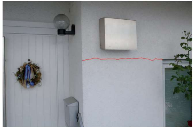
Figure A4.3.58. Thick diagonal shear crack in a modern masonry building (left); horizontal shear crack in a newer masonry building (right) induced by the 2014 Darmstadt earthquake. From Schwarz et al. (2015).
