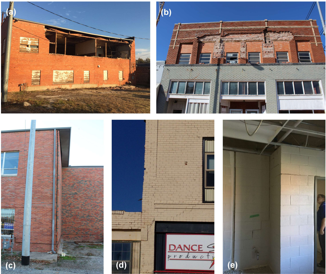
Figure A3.5.56. Examples of damage of unreinforced masonry buildings: (a) out-of-plane failure of an entire wall section of the Cushing Publishing building (not in use, photo by A. Masroor); (b) out-of-plane collapse and bulging of outer wythe (photo by E. Jampole); (c) brick façade separated from concrete masonry wall inner wythe at former St. Peter and Paul Catholic Church (photo by E. Jampole); (d) step cracks in brick wall (photo by A. Greer); (e) step cracks in concrete masonry wall (photo by E. Wilson). All photos from EERI Oklahoma USA Earthquakes Clearinghouse (2016).
