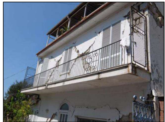
Figure A4.13.49. Diagonal shear cracks in masonry buildings. From D'Ambra et al. (2017; left) and Zuccaro et al. (2017; right).
