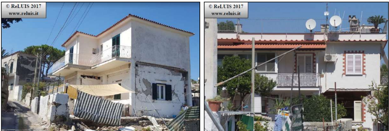
Figure A4.13.52. Detachment (left) and collapse (right) of infill panels of RC buildings. From D'Ambra et al. (2017).
