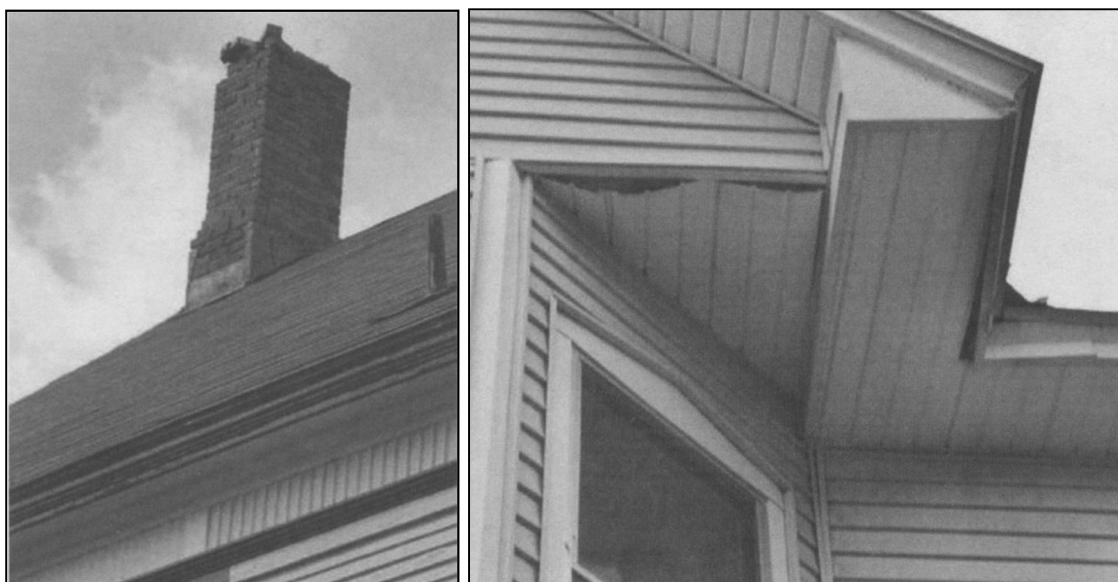
Figure A4.9.25. Rotation and partial destruction of a chimney in Au Sable Forks (left); deformed cornices at a residential building in Au Sable Forks (right). From Pierre & Lamontagne (2004).
