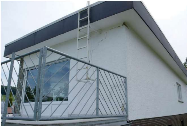
Figure A4.3.58. Thick diagonal shear crack in a modern masonry building (left); horizontal shear crack in a newer masonry building (right) induced by the 2014 Darmstadt earthquake. From Schwarz et al. (2015).
