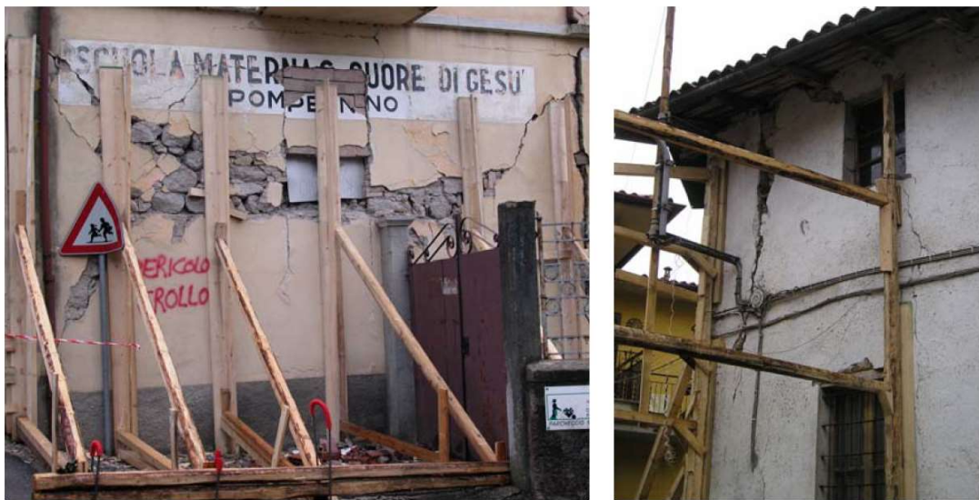
Figure A4.11.28. Collapse of masonry wall of poor quality (left) and out-of-plane deformation and cracking of masonry walls (right) in Pompegnino (MCS VII-VIII). From Dimova et al. (2004).
