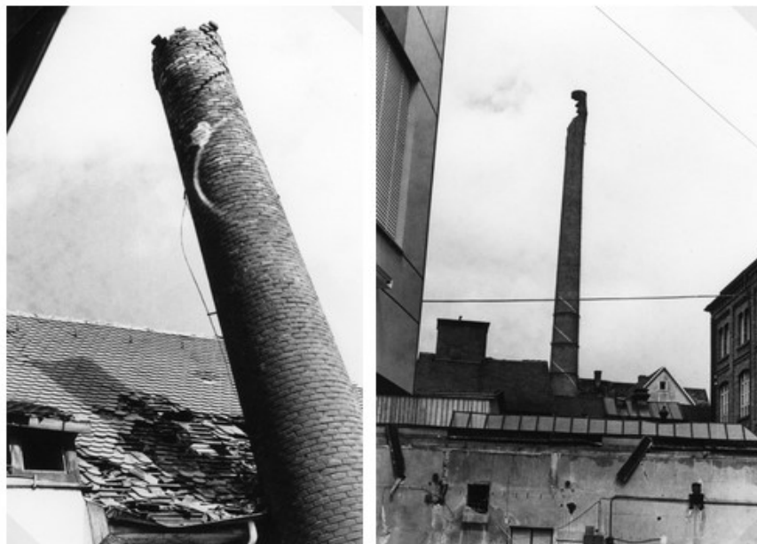
Figure A4.3.51. Damage to factory chimneys observed during the 1978 Albstadt earthquake. From Schwarzwälder Messenger (2013).
