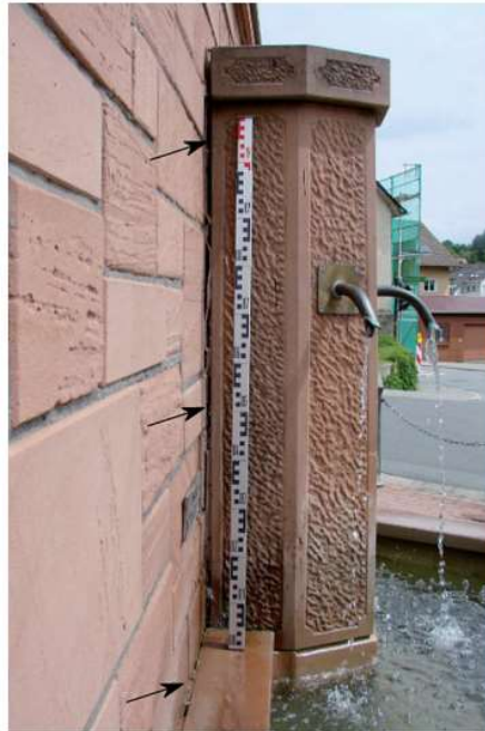
Figure A4.3.55. Rotation of the fountain up to 2.5 cm at the joint (a process which also affected many chimneys) during the 2014 Darmstadt earthquake. From Schwarz et al. (2015).
