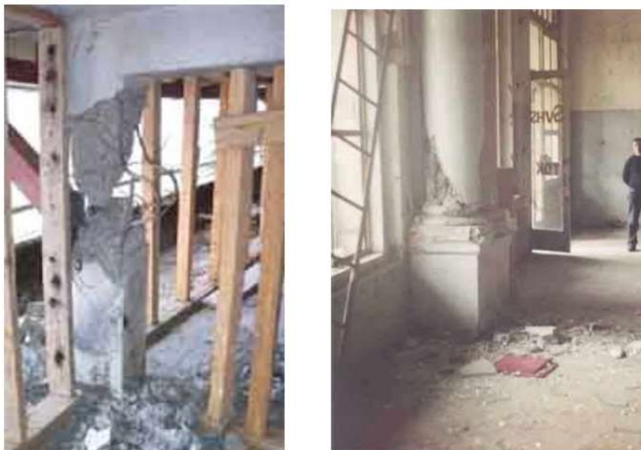
Figure A4.10.25. Damage to columns. Inst. of Mathematics (a); residential building in Kostava str. (b). From Gabrichidze et al. (2004).
