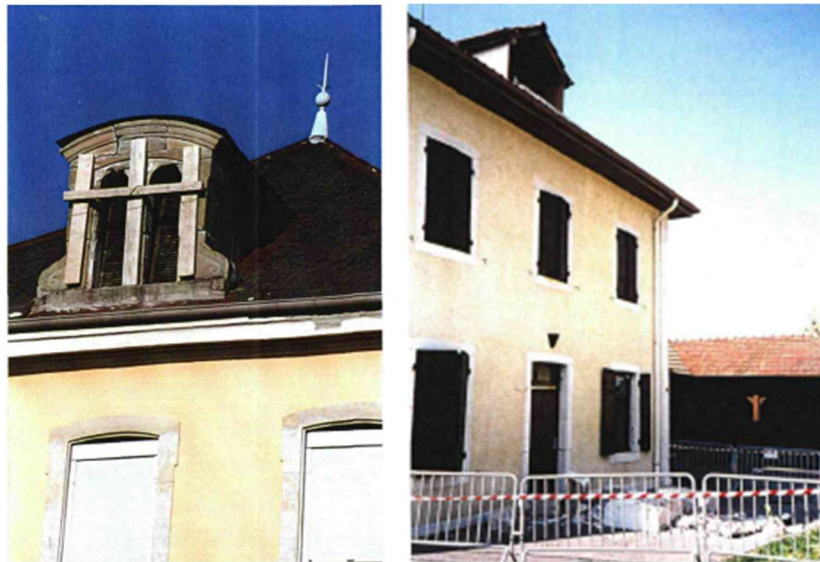
Figure A4.8.29. Confined dormer of Rumilly hospital severely cracked (left); fall of stone dormer at the nursery school of Metz-Tessy (right). From Dominique et al. (1996).
