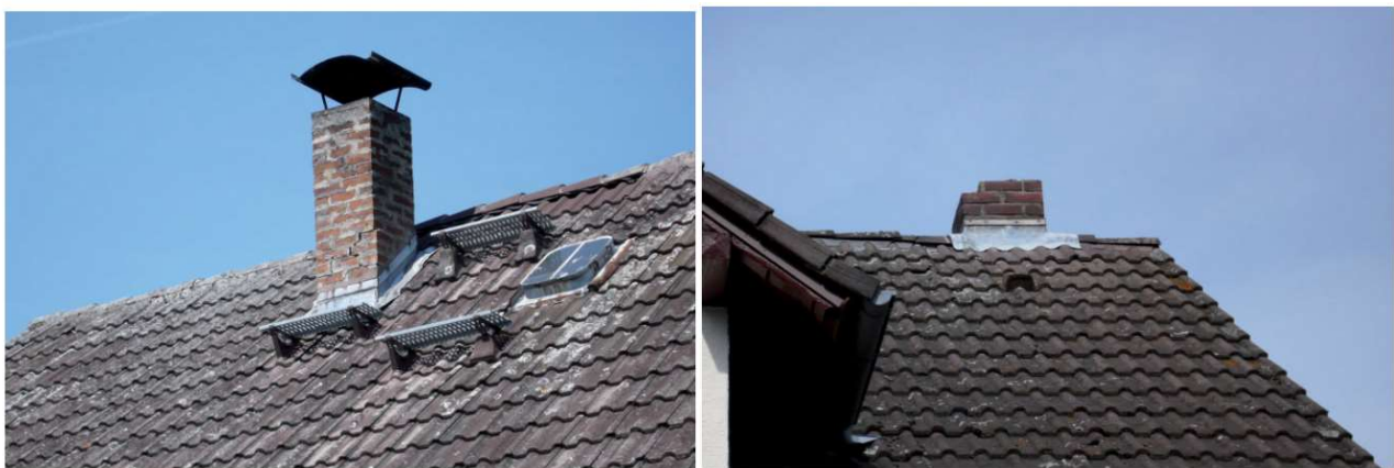
Figure A4.3.54. Cracking of a chimney stack (left) and damage to roof tiles (right) induced by the 2014 Darmstadt earthquake. From Schwarz et al. (2015).
