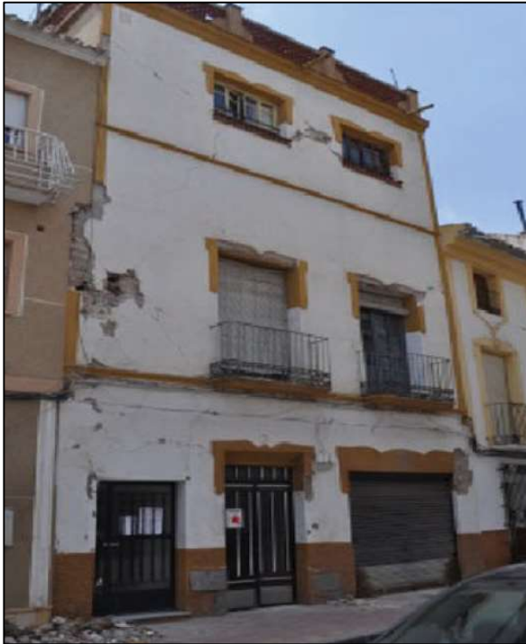
Figure A3.3.39. Examples of masonry buildings that suffered EMS-98 damage grade 3 (left) and 4 (right). From Basset-Salom & Guardiola-Víllora (2014).
