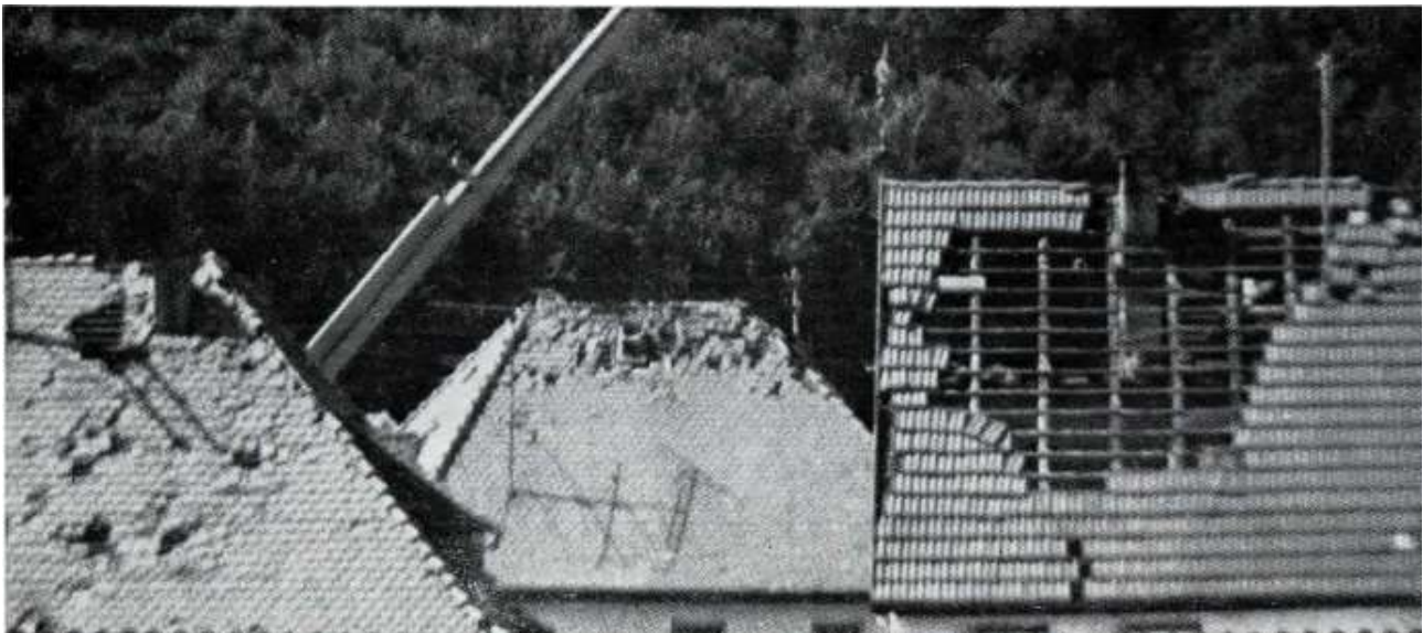
Figure A4.3.47. Falling of roof tiles induced by the 1978 Albstadt earthquake. From Blauß (1980).
