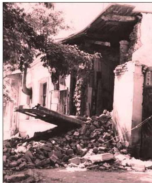
Figure A4.2.17. Damage to buildings made of crude brick. From Attention! Earthquake! (2017).
