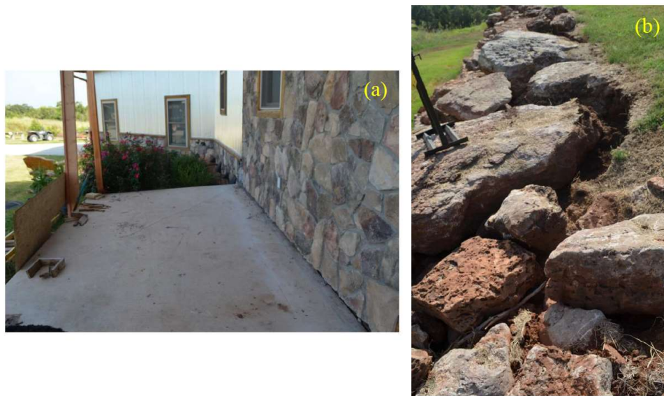
Figure A3.5.39. Porch settlement (left) and slump failure causing it (right) due to the 2016 M5.8 Pawnee earthquake. From GEER report (Clayton et al. , 2016).
