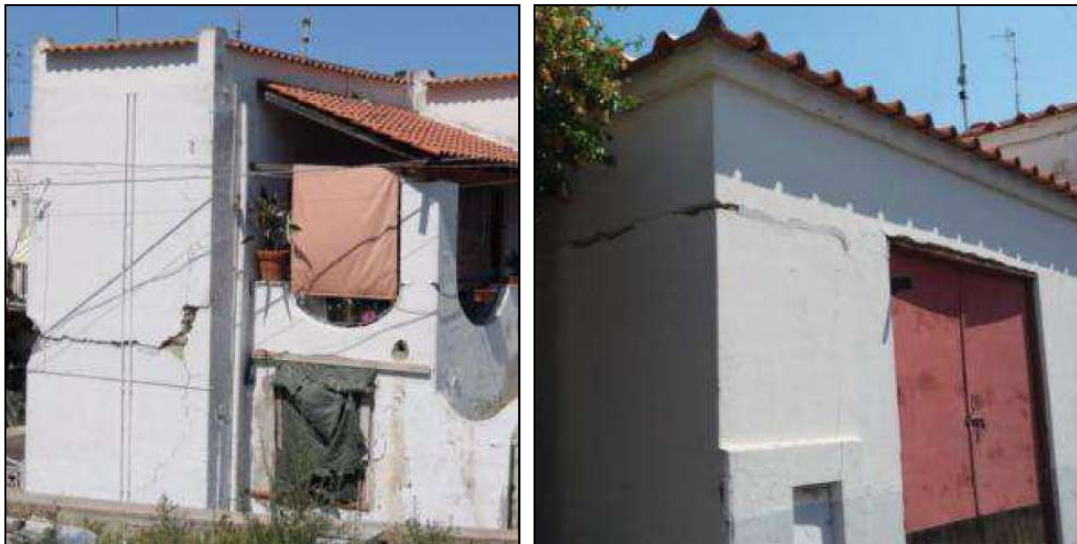
Figure A4.13.54. Horizontal crack at floor level due to story drift (Zuccaro et al. , 2017)
