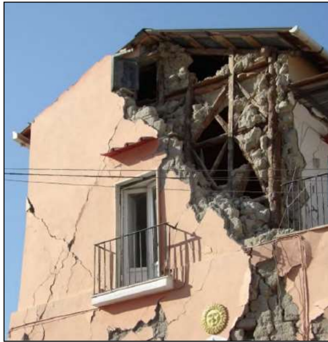
Figure A4.13.51. Damage to the masonry walls of the dual system building (Lekkas et al. , 2017).
