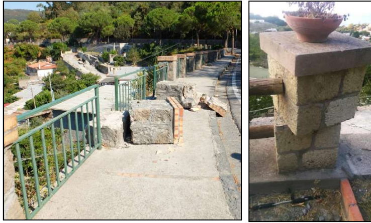
Figure A4.13.56. Collapse of parapet side walls (left) (Di Manna et al. , 2017); rotation of tuff stone column (centre) (INGV G.D.L., 2017); collapse of house retaining wall (right) (INGV G.D.L., 2017).
