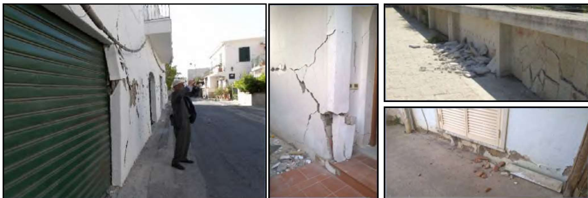
Figure A4.13.55. Damage in different buildings evidencing the impact of the high vertical seismic component (Lekkas et al. , 2017).
