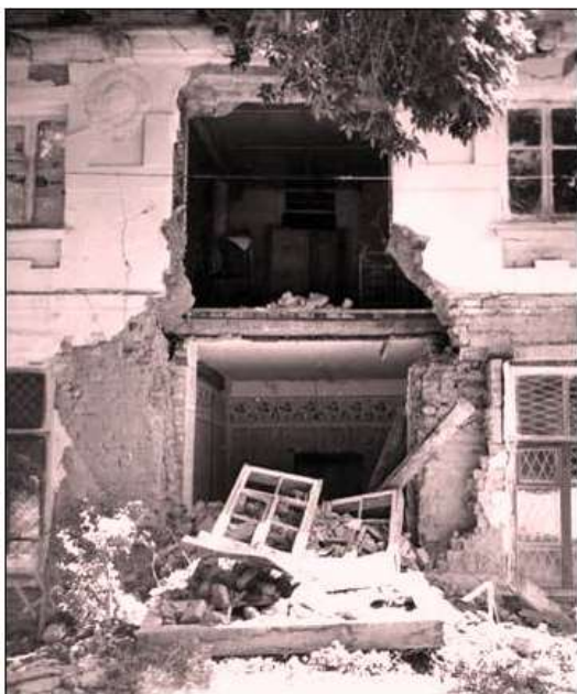
Figure A4.2.17. Damage to buildings made of crude brick. From Attention! Earthquake! (2017).
