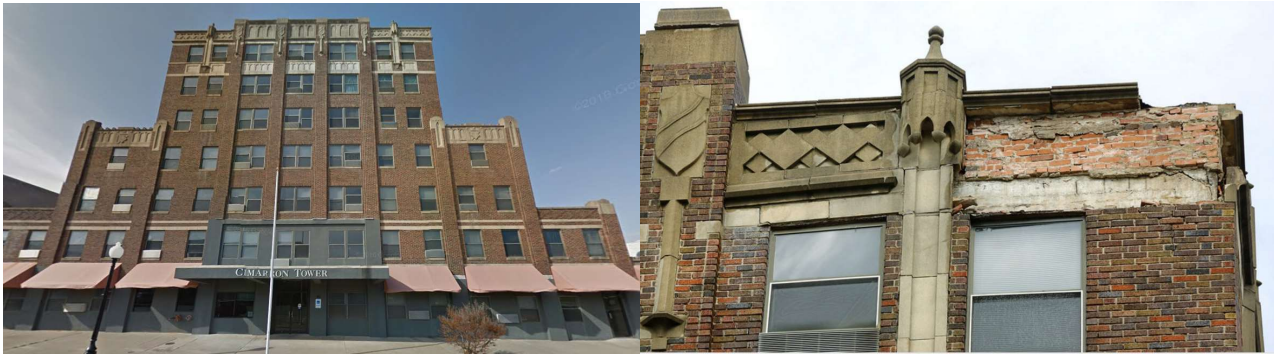
Figure A3.5.57. Damage to the roof parapet and cornices of 7-storey reinforced concrete Cimarron tower: before (left, Google Street View) and after the 2016 M 5.0 Cushing earthquake (right, photo by Jim Beckel, The Oklahoman, from News OK photo gallery, 2016g).
