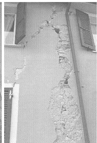
Figure A4.11.31. Fall of plaster and cracking of masonry wall in the school of Sàbbio Chiese (left), damage to infill masonry of an RC building in Clibbio (centre) and damage to load-bearing masonry in the junction between two neighbouring buildings in Salò (right). From Camassi et al. (2011; left) and Bernardini et al. (2005; centre and right).
