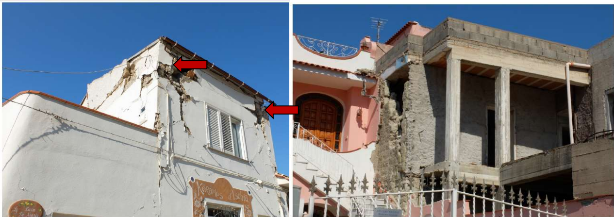
Figure A4.13.44. Masonry building with addition of steel rods under the roof (left), and enlargement of building with attempts of structural strengthening by means of RC elements (right). From Di Manna et al. (2017).
