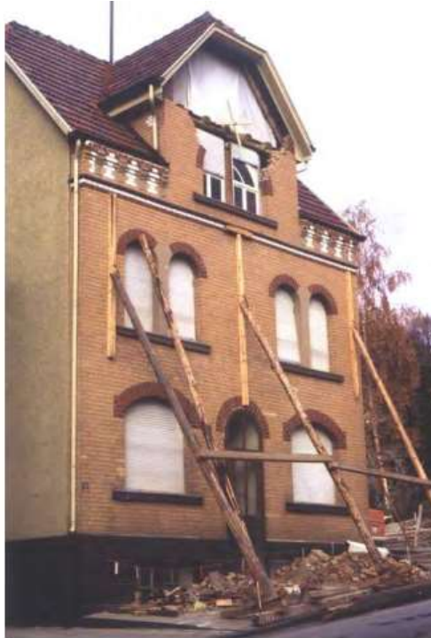
Figure A4.3.50. Damage to the gable end of a masonry building observed during the 1978 Albstadt earthquake. From Schwarz et al. (2010b)
