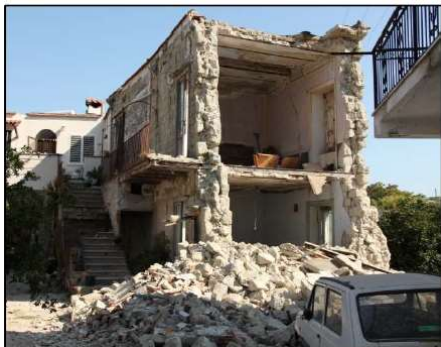
Figure A4.13.50. Out-of plane wall failure in Fango at Lacco Ameno (left); masonry expulsion and diagonal cracks in Casamicciola red zone (centre); delamination of wythes and corner failure (right). From Azzaro et al. (2017; left and centre) and Di Manna et al. (2017; right).
