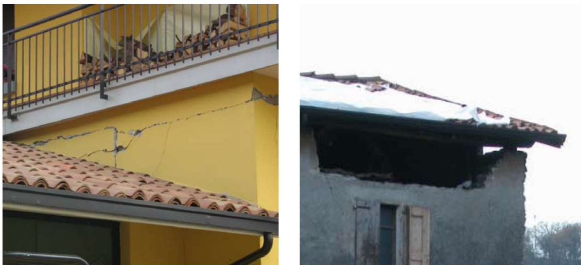
Figure A4.11.29. Failure of masonry due to pounding between buildings without seismic joints (left) and disintegration and failure of unconfined masonry under roof structures in Pompegnino (MCS VII-VIII). From Dimova et al. (2004).
