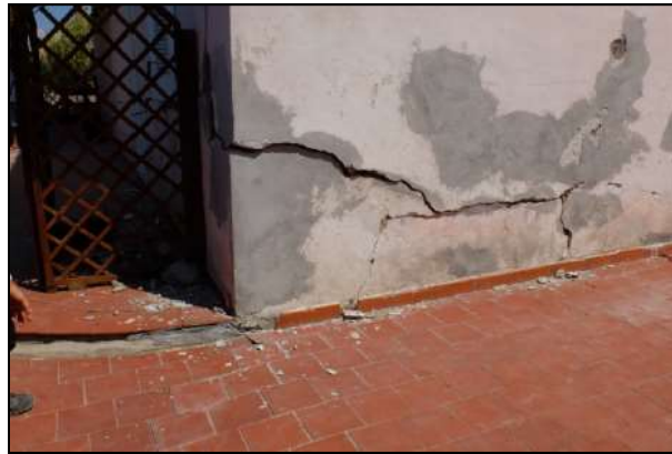
Figure A4.13.53. Subsidence of foundation of a residence in Fango (Di Manna et al. , 2017).
