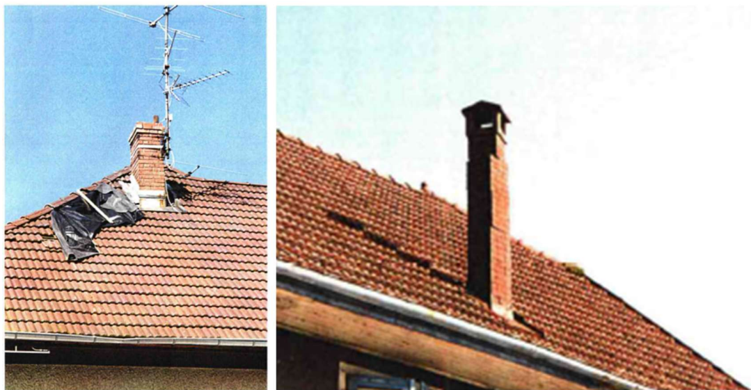
Figure A4.8.28. Damaged roof from chimney fall in Metz Tessy (left). Rotated chimney in Chaumontet (right). From Dominique et al. (1996).
