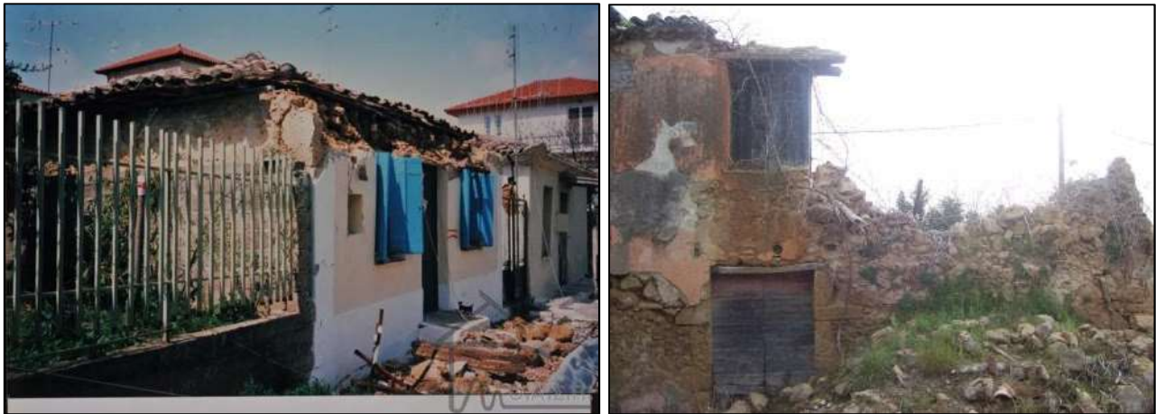
Figure A4.7.36. Adobe masonry buildings with damage from partial or total collapse (source: EPPO; left); “Motsaiko”, erected in the 19 th century, was the only building that collapsed almost completely (source: Vitinaika, 2008; right).
