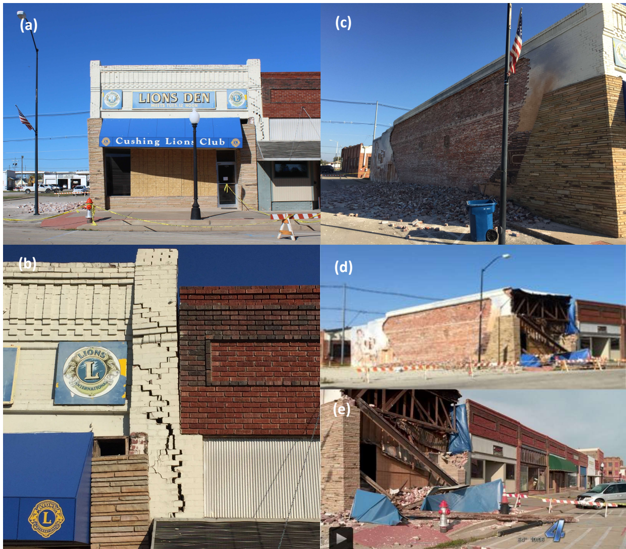
Figure A3.5.54. Damage sustained by the Lion's Den: (a) Residual deformation (photo by E. Jampole, from EERI Oklahoma USA Earthquakes Clearinghouse, 2016); (b) severe cracking in structural masonry wall (photo by A. Masroor, from EERI Oklahoma USA Earthquakes Clearinghouse, 2016); (c) failure of outer wythe of façade brickwork on side wall (photo by A. Masroor, from EERI Oklahoma USA Earthquakes Clearinghouse, 2016); (d) failure of façade in March 2017 (from 1600KUSH, 2017); (e) failure of façade in March 2017 (KFOR, 2017).
