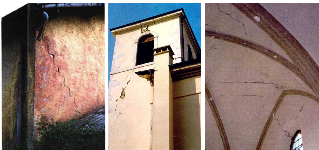
Figure A4.8.30. Deep cracks on the angle of a building in Pont-Verre (left), from Dominique et al. (1996). Large cracks on the severely damaged church of Epagny (centre) and cracks at the vault of the church in Poisy (right), both from Davidovici (N/A).
