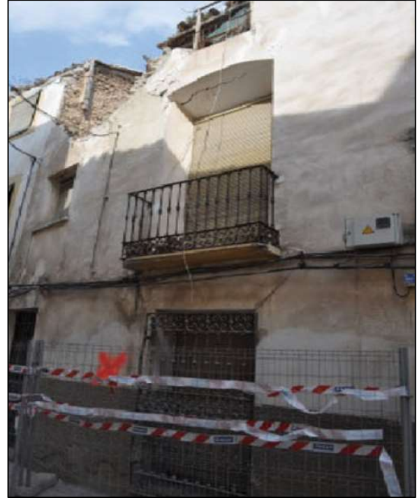
Figure A3.3.39. Examples of masonry buildings that suffered EMS-98 damage grade 3 (left) and 4 (right). From Basset-Salom & Guardiola-Víllora (2014).
