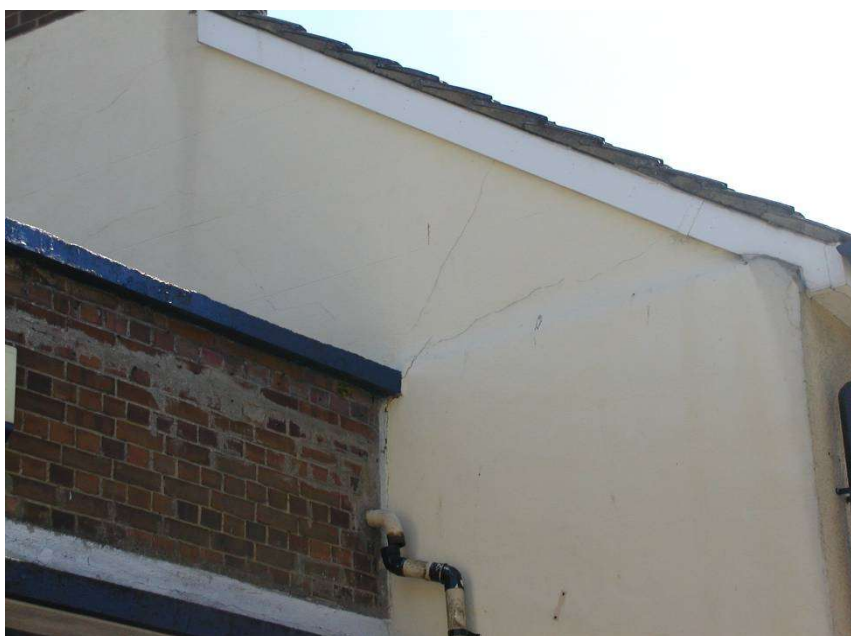
Figure A4.12.35. Cracking at junction between terrace house style (to right) and a 1960s inserted replacement property. Photograph credit: P.W. Burton, courtesy of Dr. G. Weatherill.
