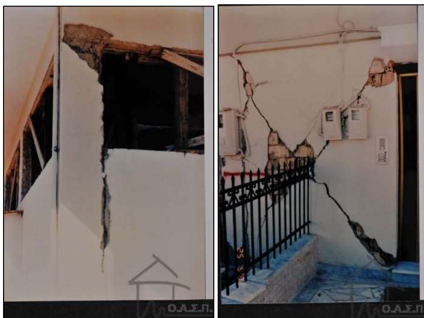
Figure A4.7.38. Example of severely damaged RC building with severe cracking and concrete spalling at the node and column and diagonal cracking of the infill panels (source: EPPO).
