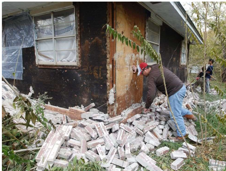
Figure A3.5.48. Façade bricks detached from the wood-frame structure of a house in Sparks. Photo by AP PHoto as in ABC News (2015).
