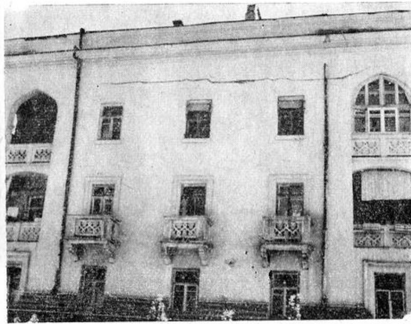
Figure A4.2.22. An example of building located in the zone of seismic intensity VIII (GOST 6249-52) with a long horizontal crack induced below the attic floor. From Rasskazovsky (1967).
