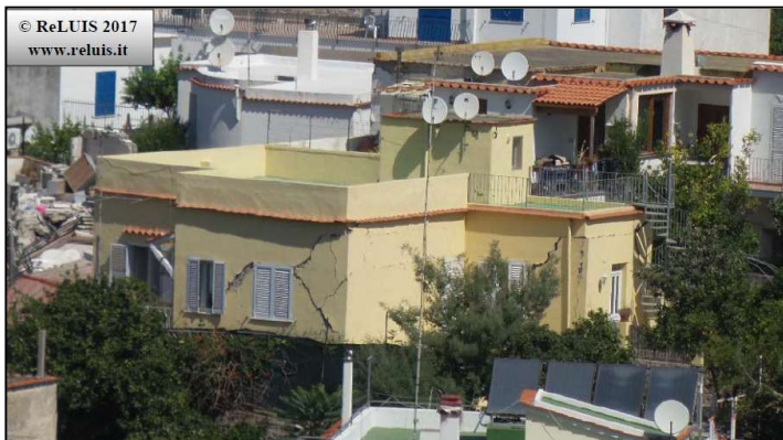
Figure A4.13.49. Diagonal shear cracks in masonry buildings. From D'Ambra et al. (2017; left) and Zuccaro et al. (2017; right).
