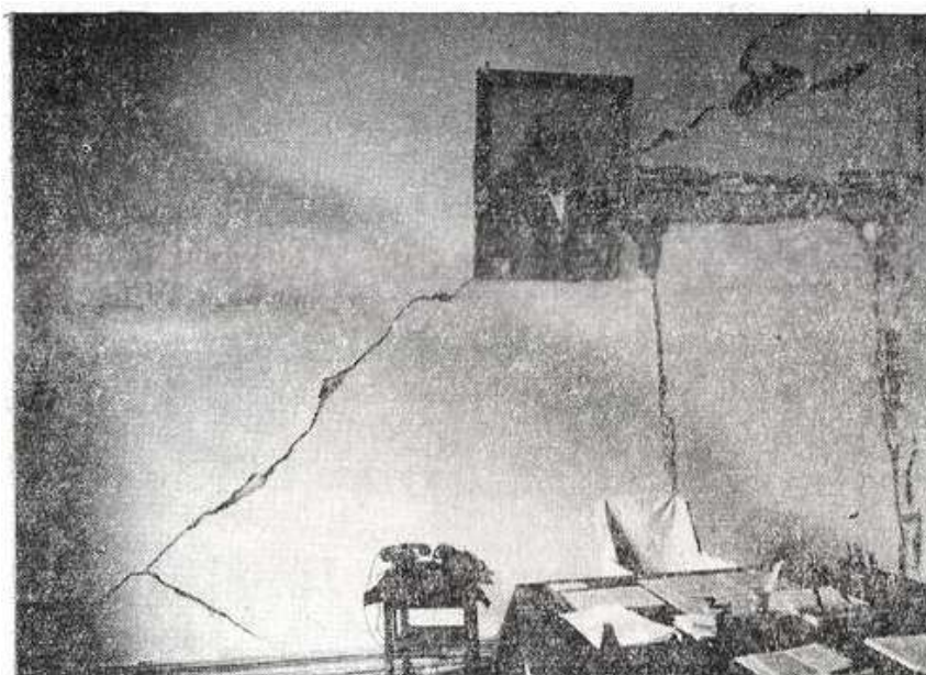
Figure A4.2.20. An example of wall cracking observed mostly in the upper floors of brick buildings located in the zone of seismic intensity VIII (GOST 6249-52). From Rasskazovsky (1967).
