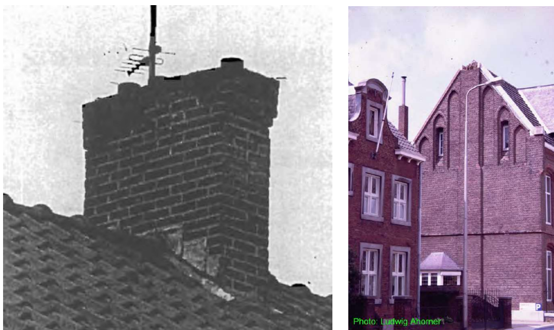
Figure A4.6.41. D2 (left) and D3 (right) damage to chimneys (Schwarz et al. , 2010).
