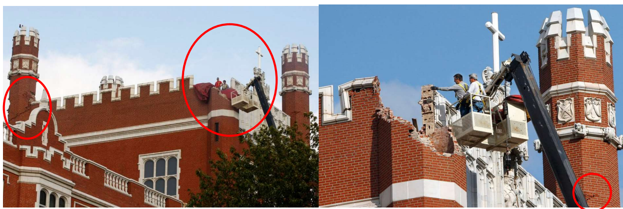
Figure A3.5.46. Damage to one of the towers of Benedictine Hall at St. Gregory's University in Shawnee after the M5.7 2011 Prague main shock. Photos by Jim Beckel, from News OK (2011).
