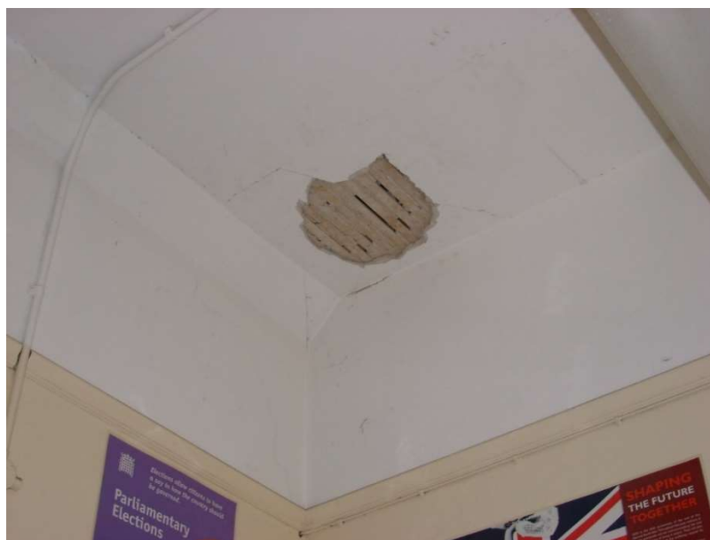
Figure A4.12.31. Harvey Boy's Grammar School: cracked and fallen plaster observed in the classroom. Courtesy of Dr. Graeme Weatherill.
