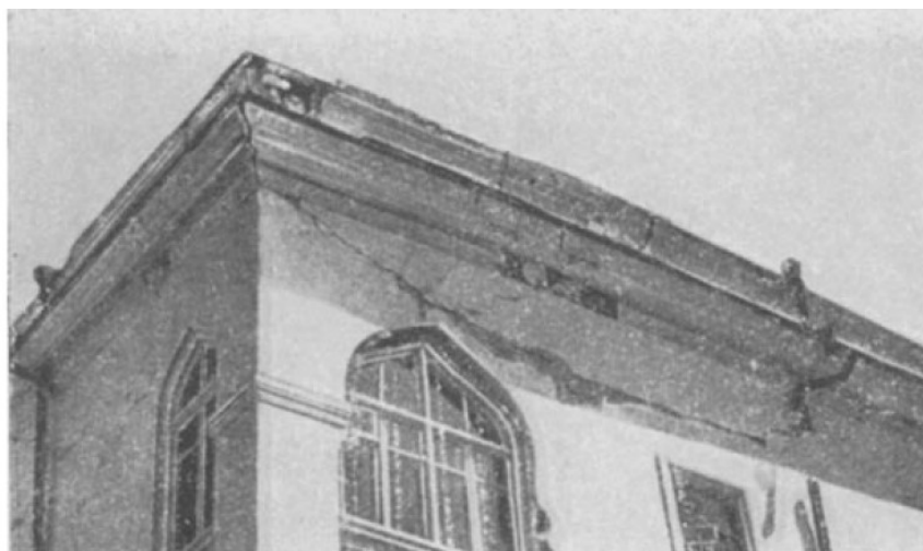
Figure A4.2.18. An example of damage induced on one of the fired brick buildings in Tashkent. From Bubis (1966).
