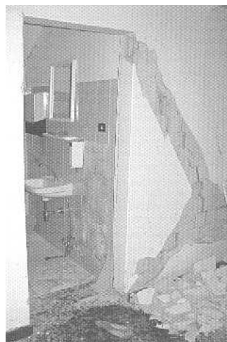
Figure A4.11.31. Fall of plaster and cracking of masonry wall in the school of Sàbbio Chiese (left), damage to infill masonry of an RC building in Clibbio (centre) and damage to load-bearing masonry in the junction between two neighbouring buildings in Salò (right). From Camassi et al. (2011; left) and Bernardini et al. (2005; centre and right).
