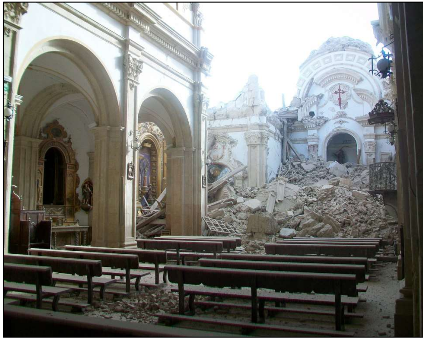
Figure A3.3.40. Collapse of the transept area of the Church of Santiago (Wikipedia).
