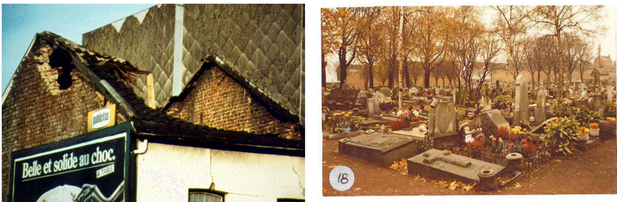
Figure A4.4.33. Roof collapse due to walls displacement, from Doneux et al. (2003) (left); cemetery of St Gilles, from EEFIT (1984) (right).
