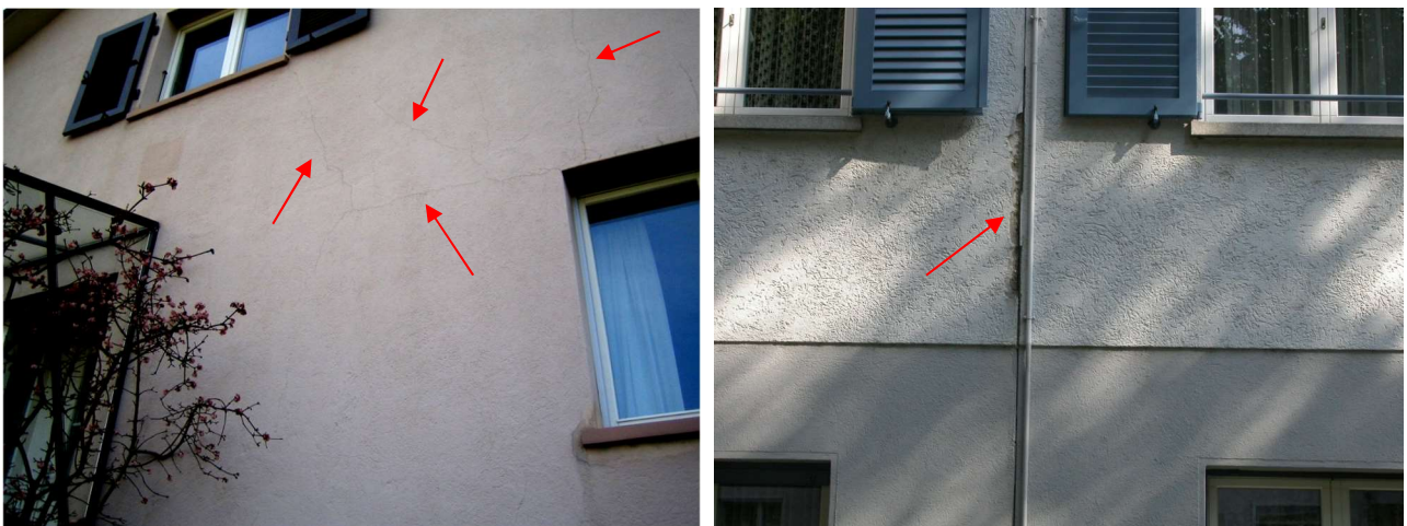
Figure A3.1.33. Hairline cracks in plaster (left). Minor plaster spalling (right).
