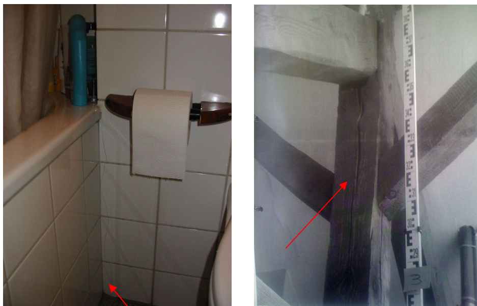
Figure A3.1.34. Crack in intersection of two perpendicular masonry elements (left). Crack parallel to the orientation of fibres in a timber element (right).
