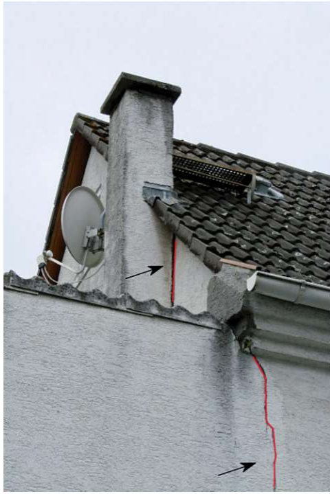
Figure A4.3.57. Cracking observed at connections between different building elements(left) and balustrade crack (right) caused by the 2014 Darmstadt earthquake. From Schwarz et al. (2015).
