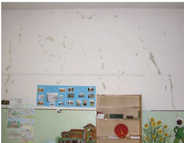
Figure A4.11.31. Fall of plaster and cracking of masonry wall in the school of Sàbbio Chiese (left), damage to infill masonry of an RC building in Clibbio (centre) and damage to load-bearing masonry in the junction between two neighbouring buildings in Salò (right). From Camassi et al. (2011; left) and Bernardini et al. (2005; centre and right).
