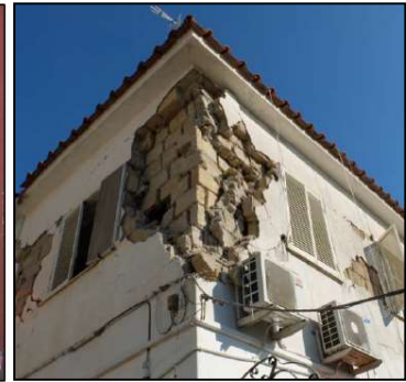
Figure A4.13.50. Out-of plane wall failure in Fango at Lacco Ameno (left); masonry expulsion and diagonal cracks in Casamicciola red zone (centre); delamination of wythes and corner failure (right). From Azzaro et al. (2017; left and centre) and Di Manna et al. (2017; right).
