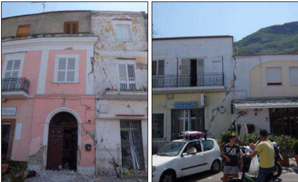
Figure A4.13.57. Damage to adjacent buildings due to hammering (Zuccaro et al. , 2017)
