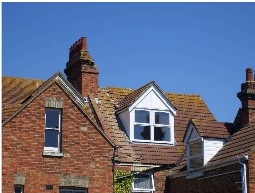
Figure A4.12.33. Chimney stack and damage to roof tiles. Photograph credit: G. Weatherill. From Sargeant et al. (2008), colour version courtesy of Dr. Graeme Weatherill.
