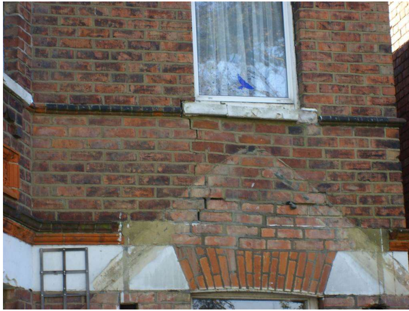
Figure A4.12.32. Cracks in masonry observed in Radnor Park Road. Photograph credit: G. Weatherill. From Sargeant et al. (2008), colour version courtesy of Dr. Graeme Weatherill.
