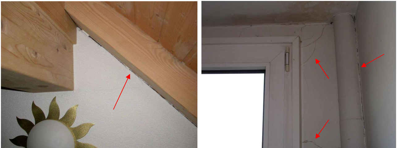
Figure A3.1.32. Crack in connection between wall and timber roof (left). Cracks in corner of a window (right).
