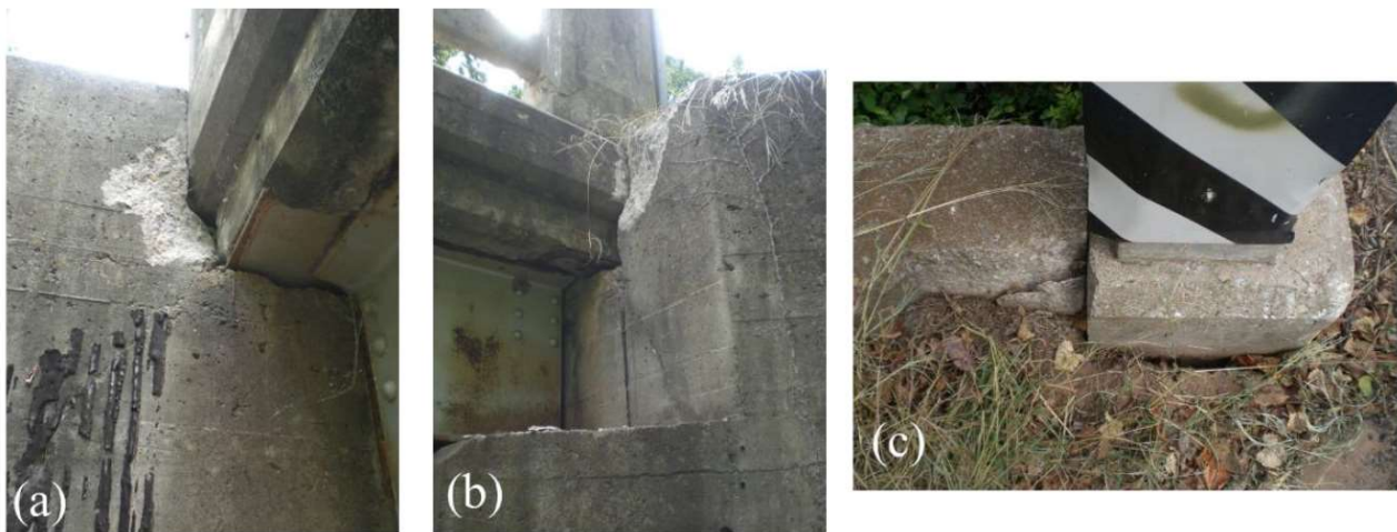
Figure A3.5.50. Damage at the west abutment of Belford Bridge, which may be due to the 2016 M5.8 Pawnee earthquake: spalling of concrete (left and centre) and 4-cm wide gap between backfill soil and abutment. From GEER report (Clayton et al. , 2016).
