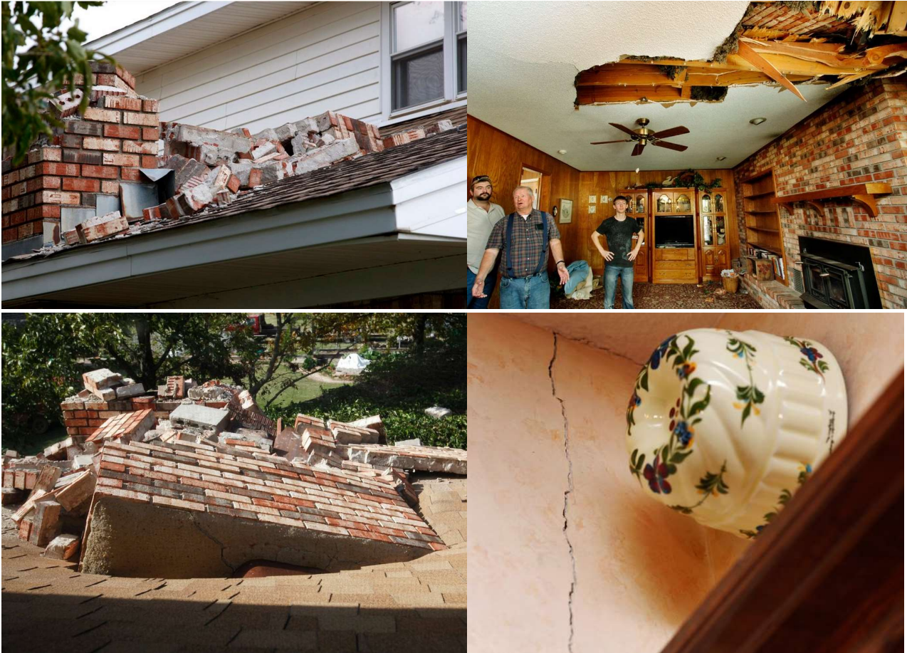
Figure A3.5.47. Damage to a house in Sparks. The chimney toppled over the roof. Photos by Sue Ogrocki (News OK, 2011).
