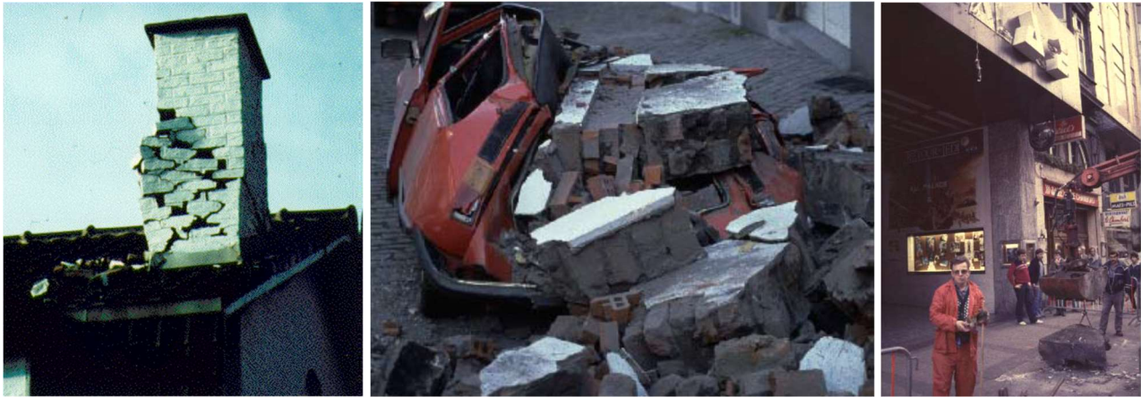
Figure A4.4.31. Chimney of good quality damaged (left); fall of chimney over a car (centre); fall of massive stone in a central road (right). From Doneux et al. (2003).
