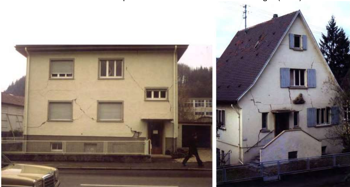
Figure A4.3.49. Extensive cracking observed at the corners of windows and doors due to the 1978 Albstadt earthquake. From Schwarz et al. (2010b).
