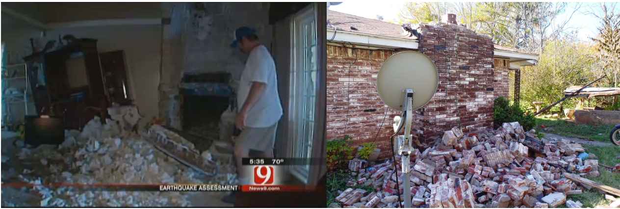
Figure A3.5.59. Complete collapse of a fireplace in the interior of a house in Sparks (left, News 9, 2011), and collapse of the top of a chimney of a house (right, Wikipedia).
