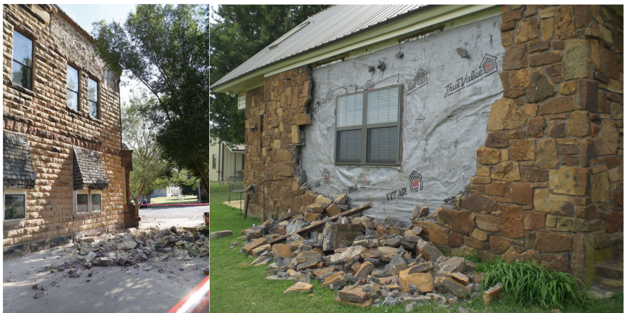
Figure A3.5.52. Examples of failures of stone façades: Arkansas Valley National Bank building (left, photo by Paul Hellstern, The Oklahoman, available from News OK (2016a), and a single-family residential house (right, photo from GEER report, Clayton et al. , 2016).
