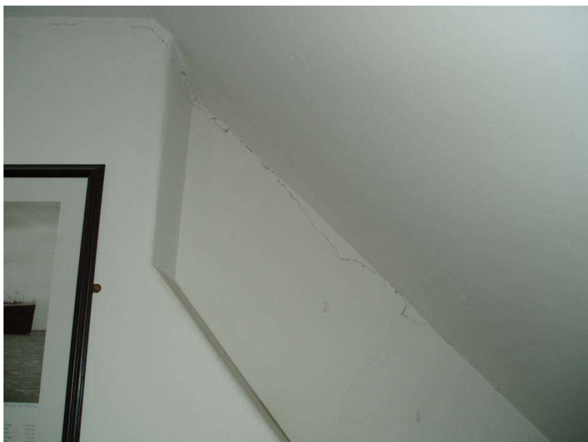
Figure A4.12.34. Cracking of interior of property in Gladstone Road. Photograph credit: S.L. Sargeant, courtesy of Dr. G. Weatherill.
