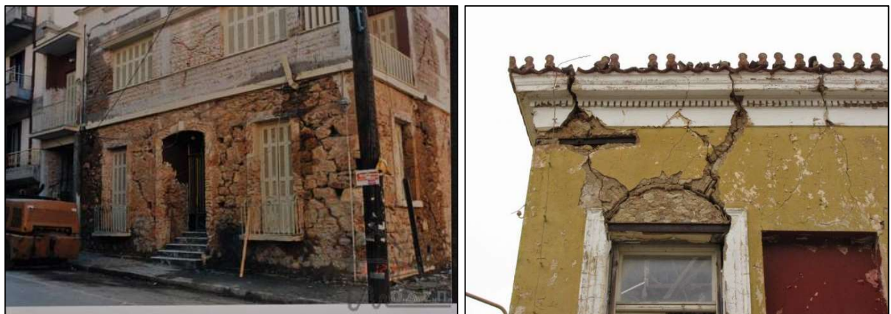
Figure A4.7.37. Severe damage to stone buildings: (left) diagonal cracking at piers (source: EPPO); (right) vertical cracking of spandrels of upper floor (source: Tempo24, 2016).
