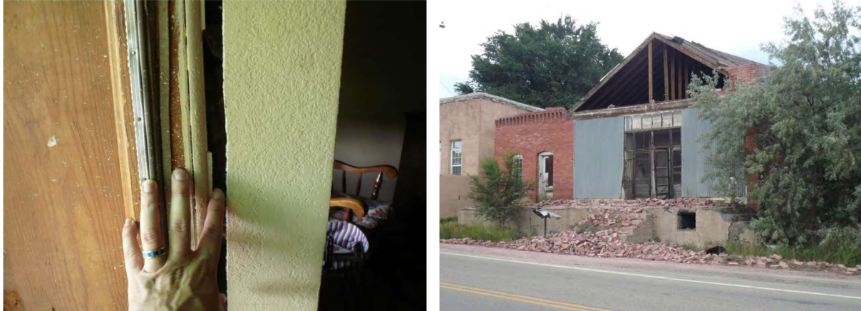
Figure A3.4.19. Damage observed at Segundo: on the left, the exterior wall pulled away approximately 2.5 cm from the interior wall; on the right, the front of this brick building collapsed (Morgan & Morgan, 2011).
