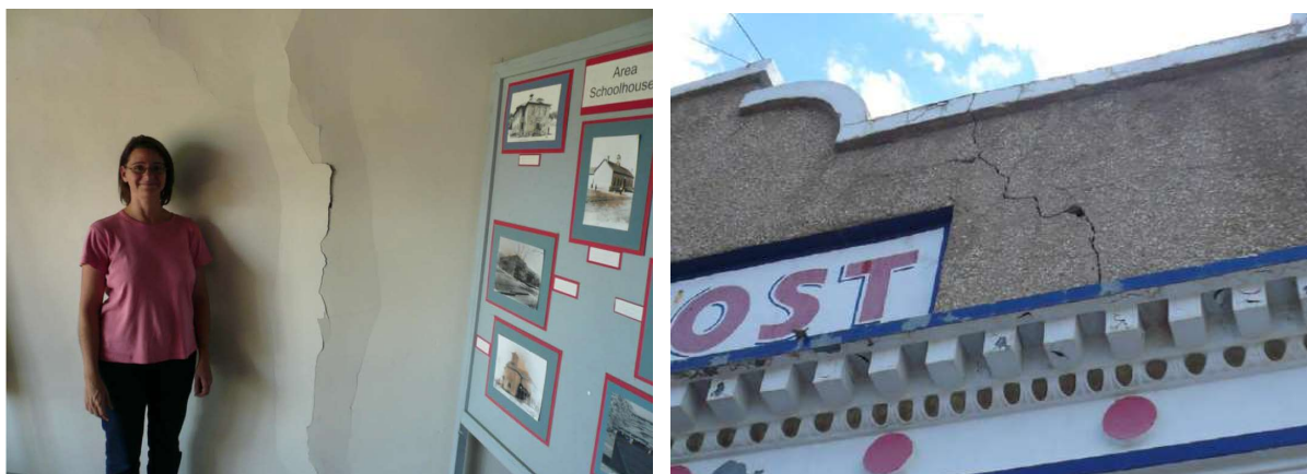
Figure A3.4.21. A 3 metres long vertical crack in the building of the Cokedale post office/city hall (left); cracked plaster on a façade in Segundo (Morgan & Morgan, 2011).
