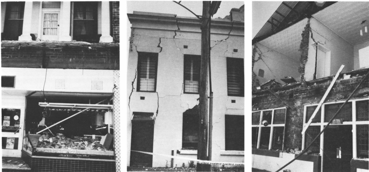
Figure A4.5.30. Awning collapse due to parapet falling onto it (left), typical damage in masonry walls (centre) and failure of both inner and outer masonry wythes of top storey and gable (right). Photos by M. Maloy, from McCue (1990a).
