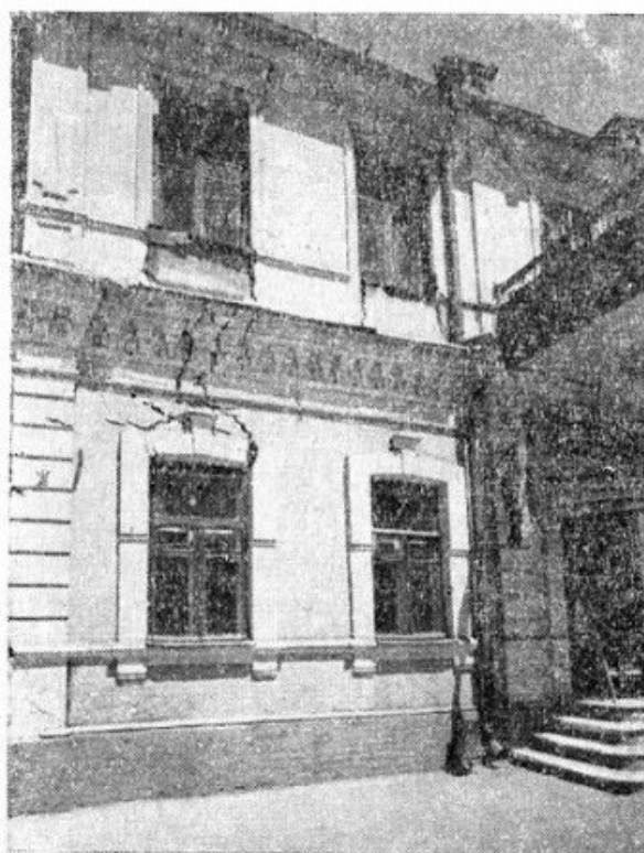
Figure A4.2.21. An example of masonry cracking commonly observed in buildings located in the zone of seismic intensity VIII (GOST 6249-52). From Rasskazovsky (1967).
